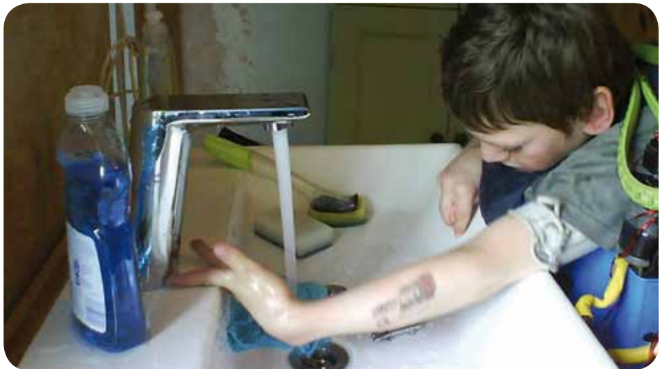
Cameron making use of the electronic sensor tap. The kitchen sink is fitted with special wall brackets and a handle so it can be manually moved up and down.
